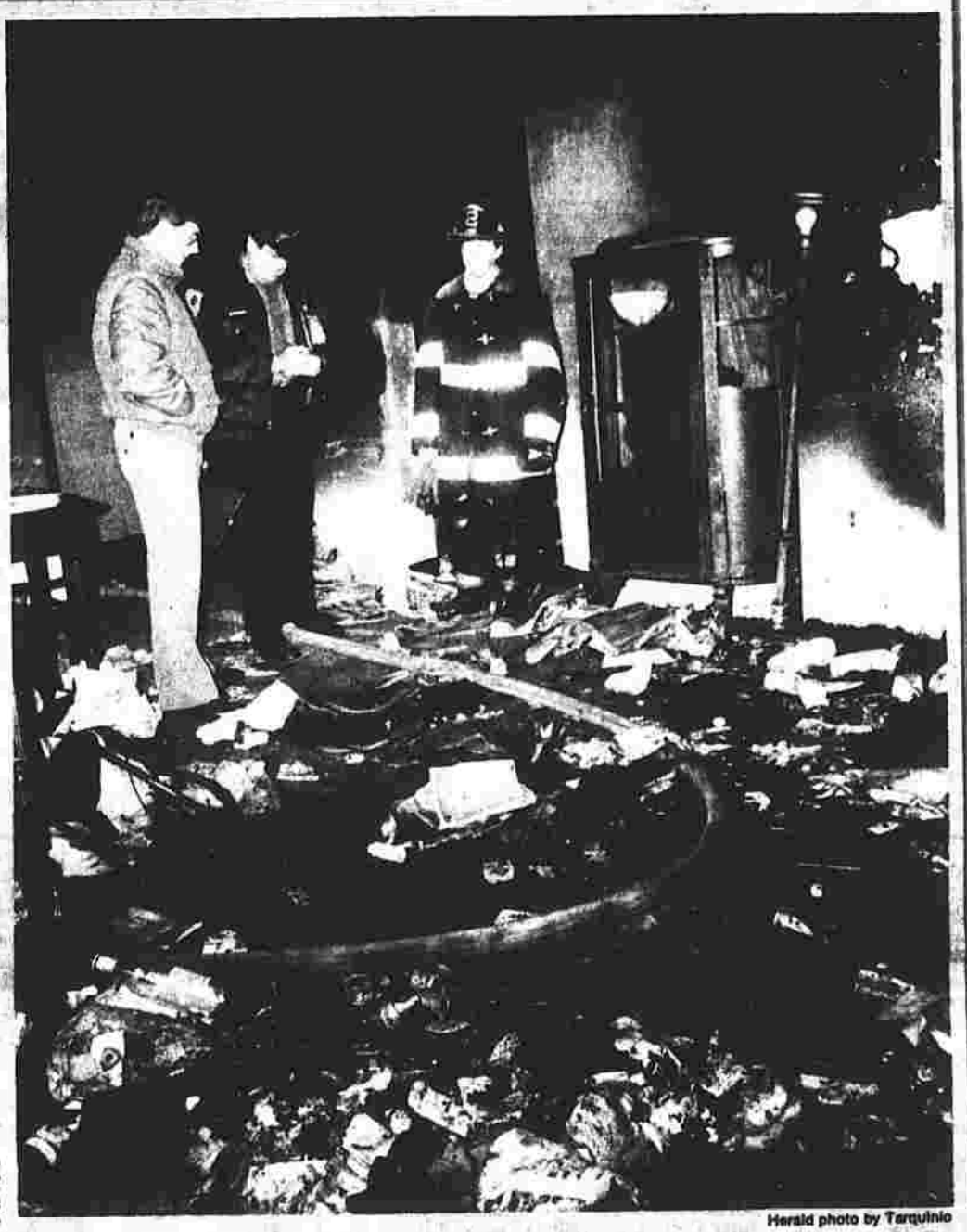
Police and fire officials inspect the damage after a fire Tuesday afternoon in an apartment at 436 North Main St. The tenant suffered burns during the blaze and was listed in critical condition at Hartford Hospital.
